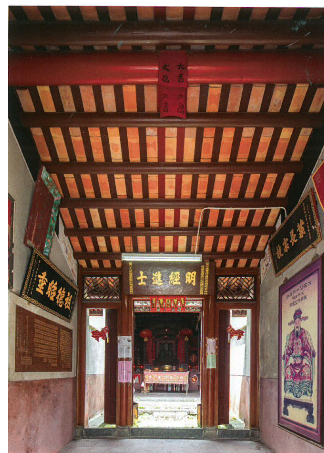
The front hall's roof of Ip Ancestral Hall has been restored, including the main ridge, gable ridges and fascia boards
