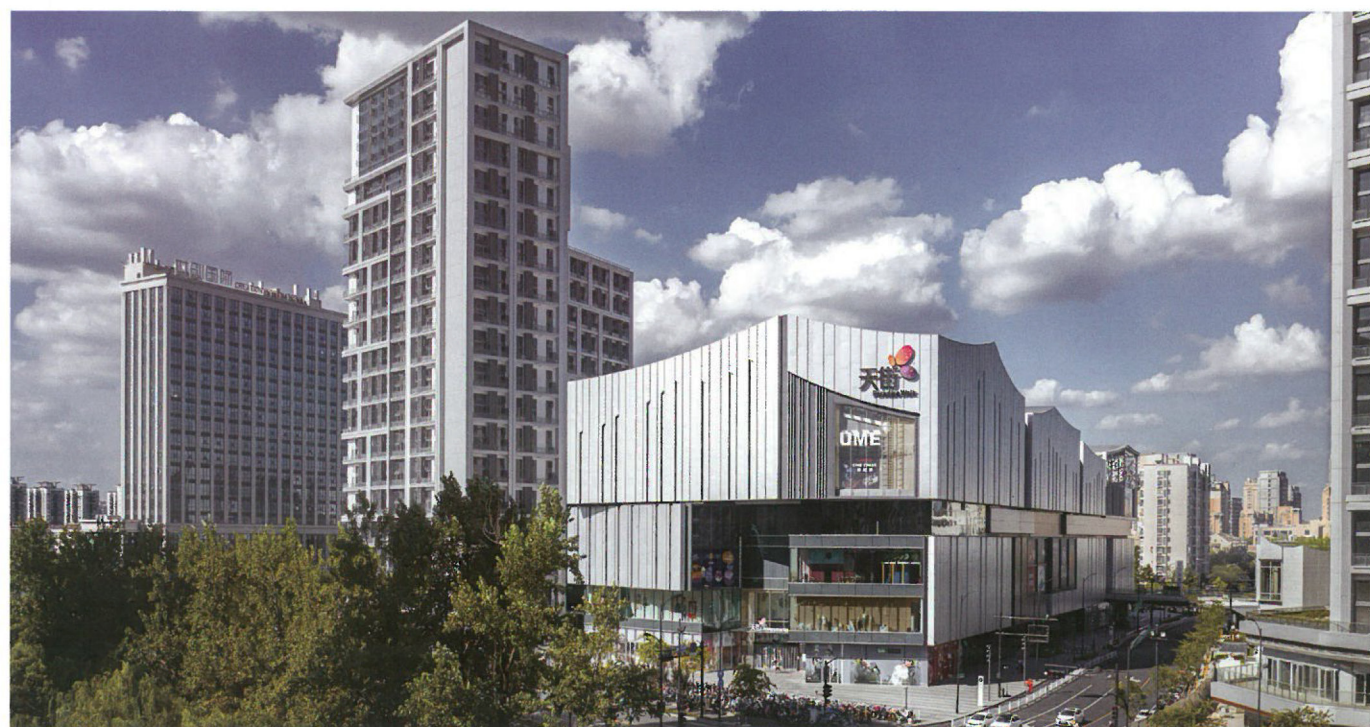
Facade material is dominated with extra-thin aluminium panels
