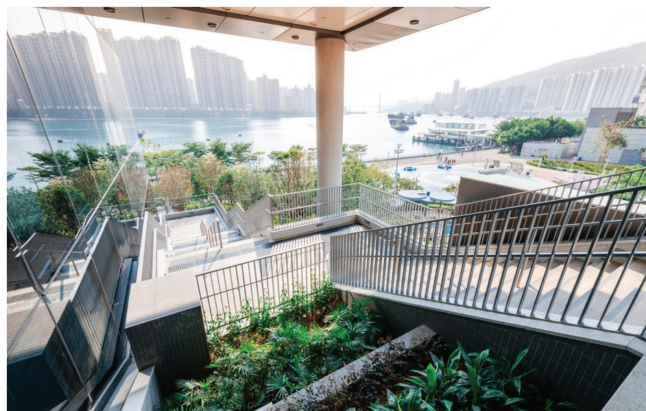
Stairs form a key architectural feature at Tsuen Wan Sports Centre, Hong Kong, China designed by LWK + PARTNERS for the scenic harbour view
