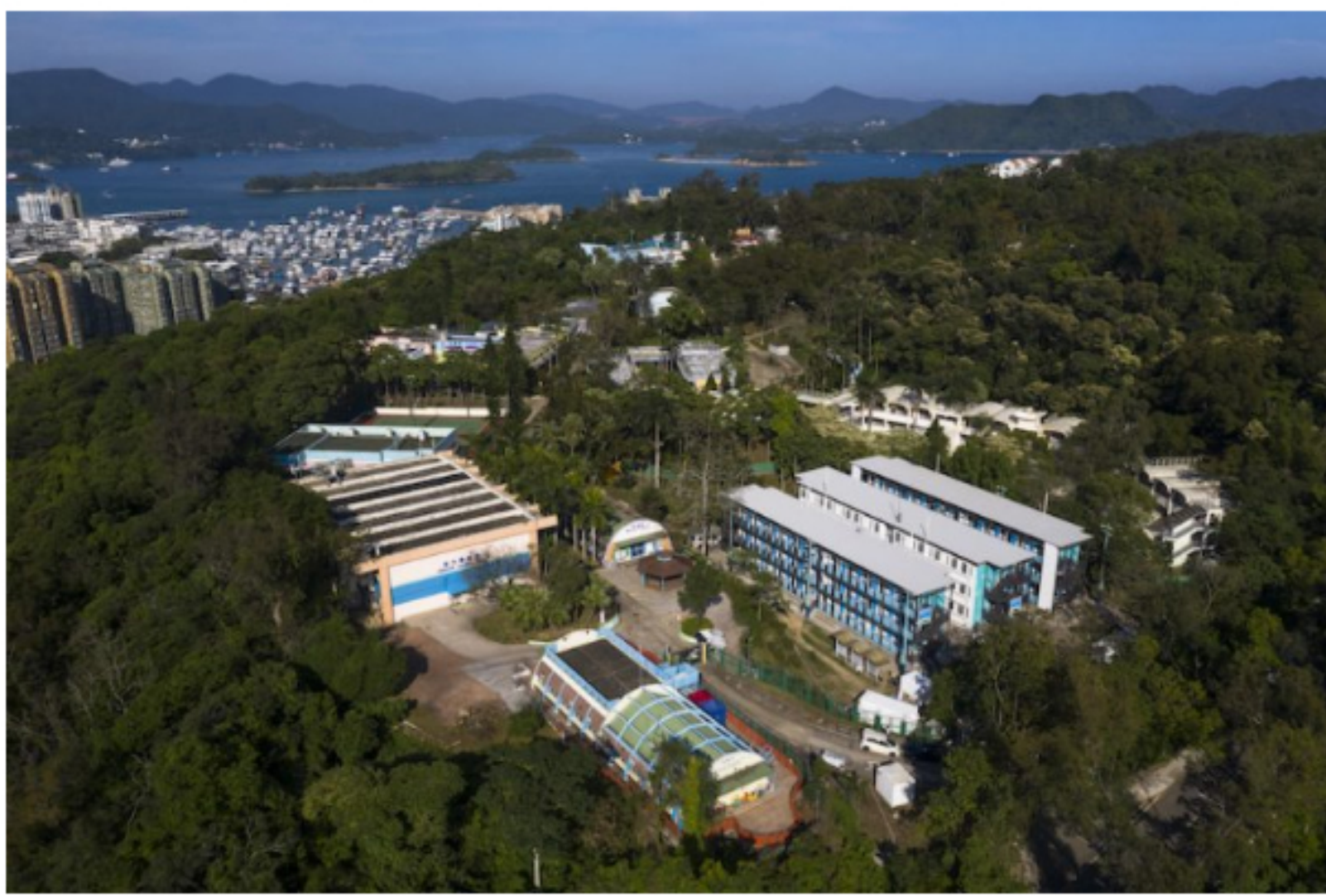
Sai Kung Outdoor Recreation Centre Temporary Quarantine Facilities, Hong Kong (Photo credit: Paul Y. - iMax)
